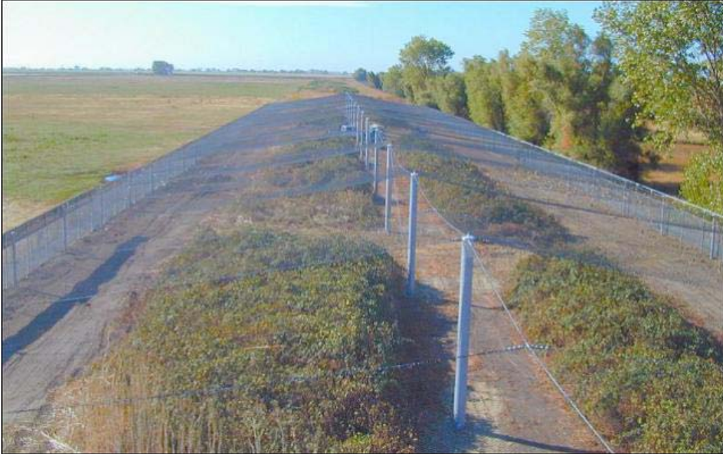
Figure 2. Photo of a portion of a pen for controlled propagation of riparian brush rabbits at Pond 6. The pen is approximately 530 feet long, 100 feet wide, and the side fencing is about 7 feet high. The top is covered with netting to prevent raptors from entering. Sides are topped with sheet metal, shown on the left, but not yet installed on the right. For scale, two vehicles are parked near the centerline (photo by L.P. Hamilton).
