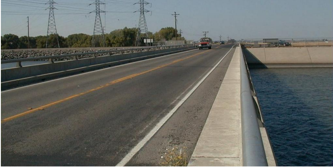
Figure 19. Highway 33 bridge over the California Aqueduct, Santa Nella, California.
