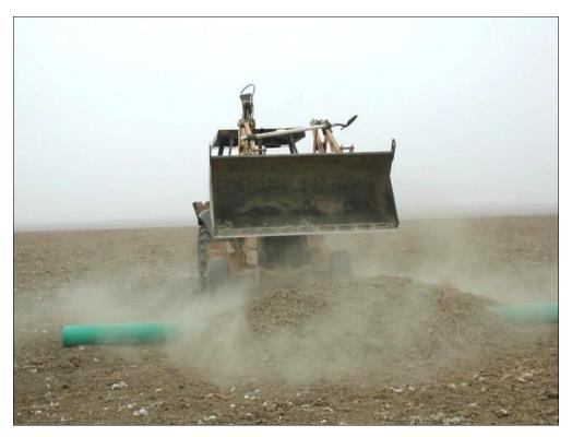
Figure 4. Double-entrance surface den being installed on Paramount Farming Company property in Kern County, California.
